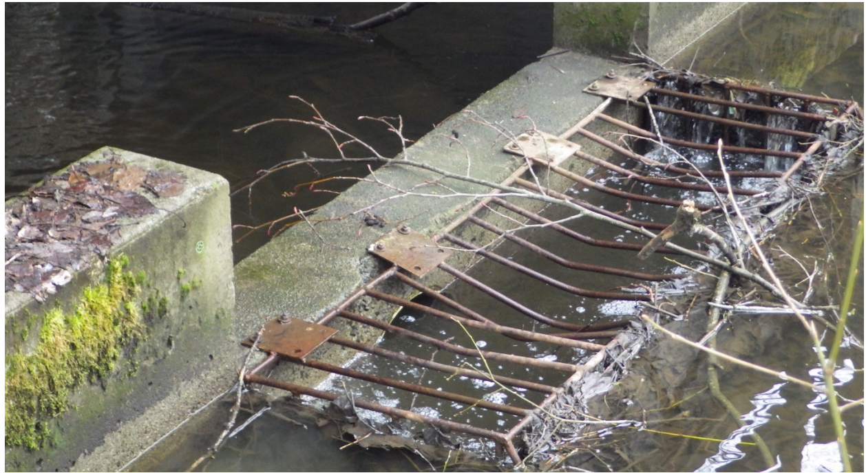
Photo 17: View of the concrete apron and debris rack at the Bon Accord Lake outlet.
