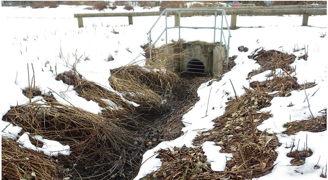
Photo 4: View of Hawthorne Creek, downstream of the BC Hydro ROW pedestrian trail and culvert, facing west.
