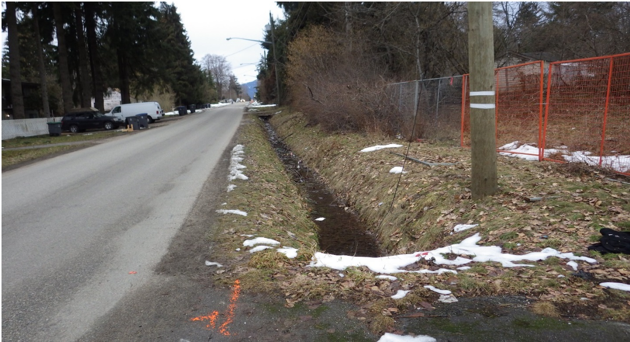
Photo 1: View of 139 Street east ditch (Class C) near proposed new road alignment, facing north.
