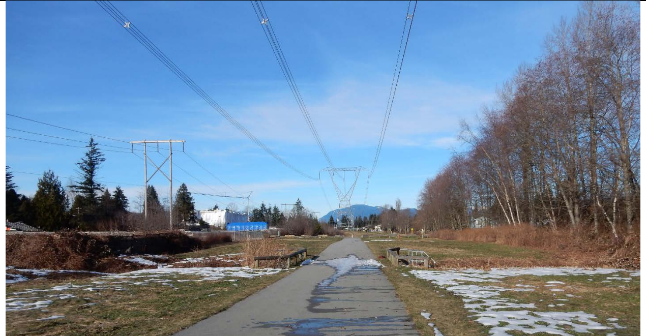
Photo 1: View of BC Hydro ROW facing north.
