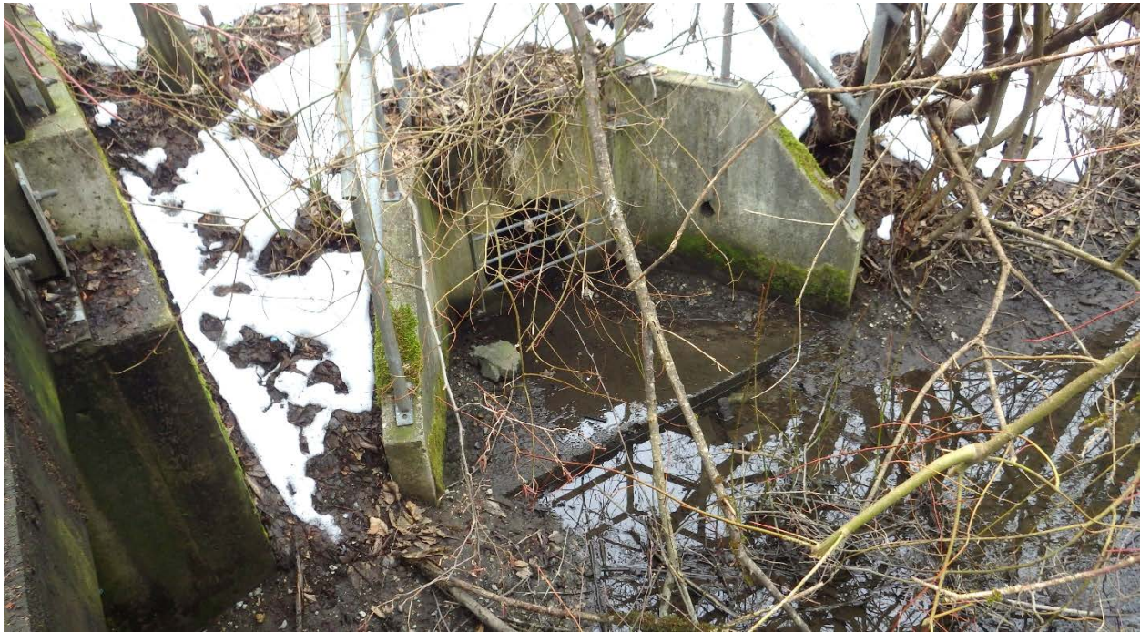
Photo 8: View of (one of seven) concrete culvert on Hawthorne Creek long 106A Avenue.
